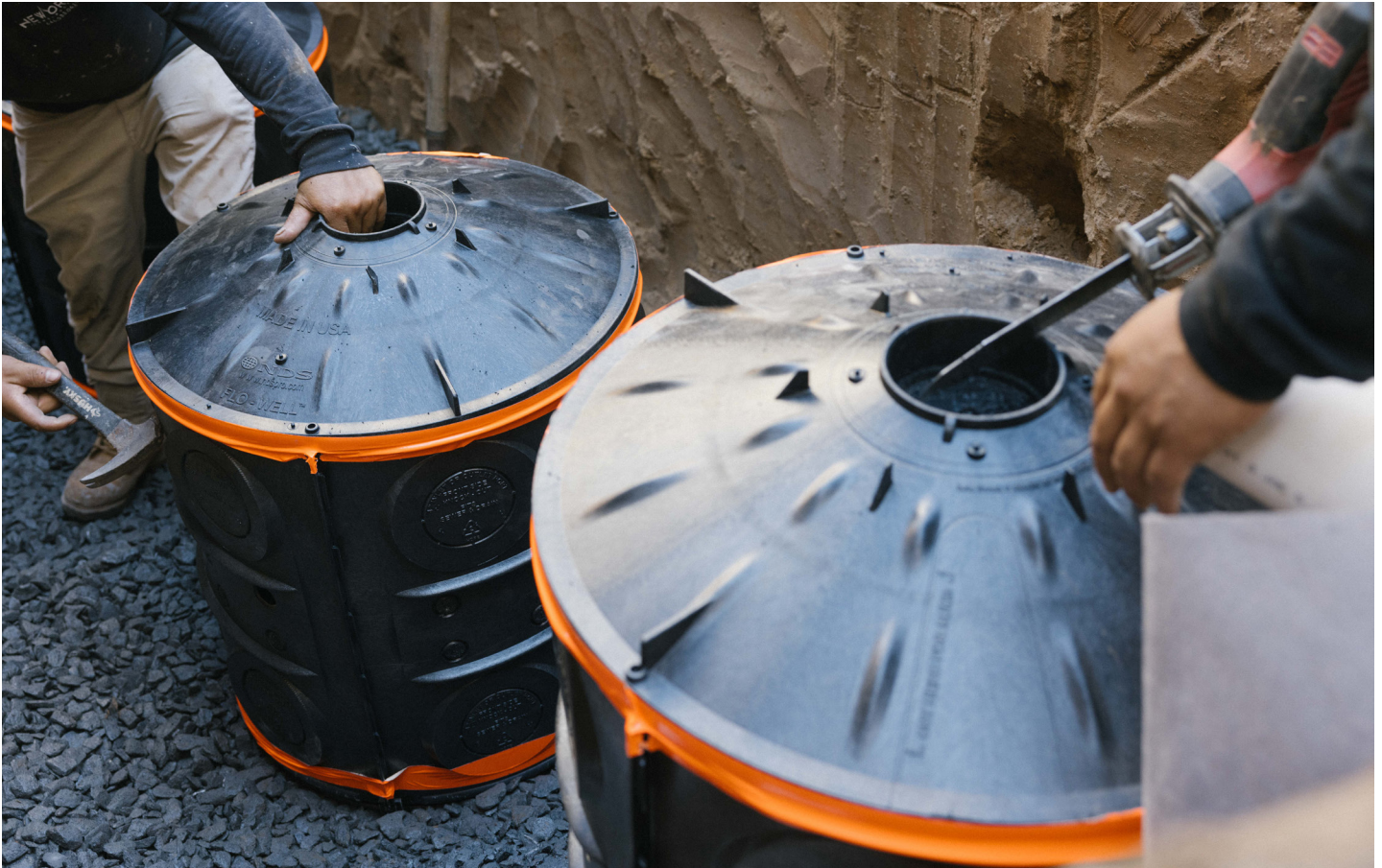
Drywells being installed at one of the 10th Street properties
